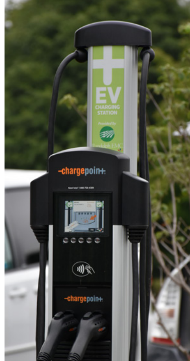
One of four new Level 2 EV charging stations at the NC Zoo provided by Randolph EMC and ChargePoint
