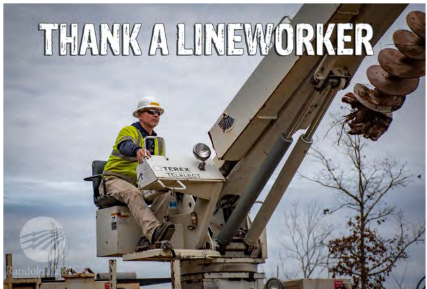
Journeyman Lineman/Foreman Rodney Haithcock works to restore power in Moore County.
