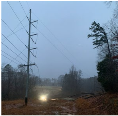
Storm damage from the Jan. 3, 2022 winter weather event
